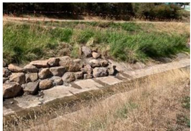
Rockwork lining in progress
